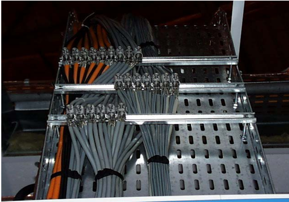
Figure 9.4 Spring clips installed on cables
