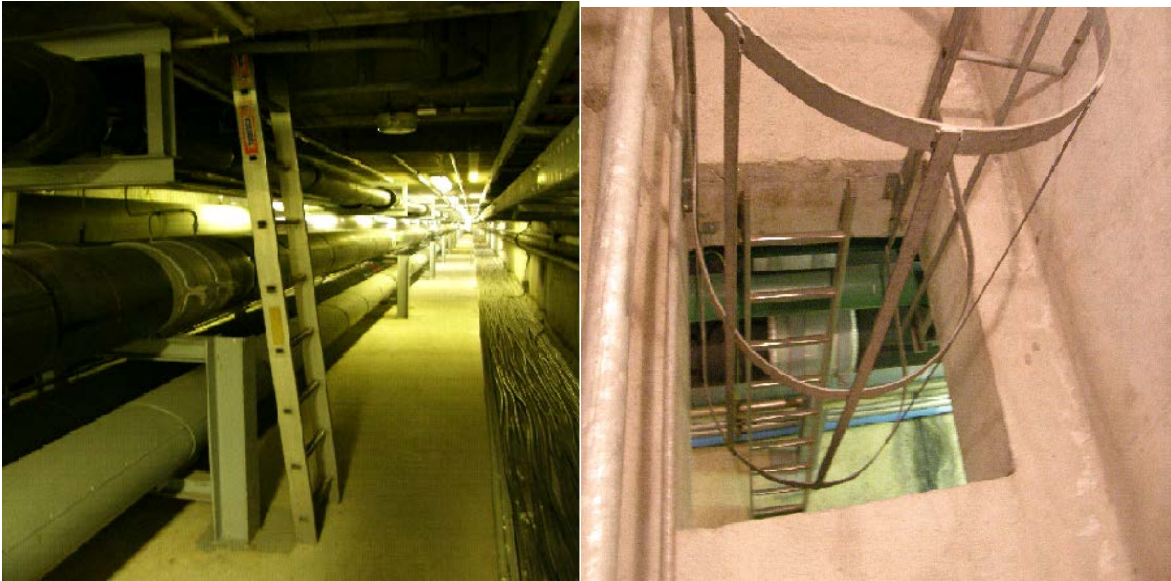
Figure 5.7.3 Manhole access from the outside to the technical gallery
